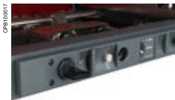
“Disconnected” position locking by keylock.
