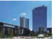
Beijing FA Center MITSUBISHI ELECTRIC AUTOMATION (CHINA)LTD.
